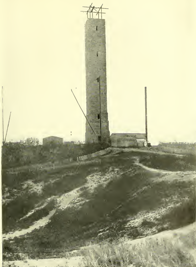
THE PILGRIM MONUMENT IN CONSTRUCTION.
